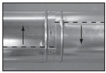
Figure 7.7 Rotate Seams for Disassembly
