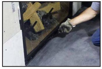
Figure 11.8. Securing Bottom Glass Clips
