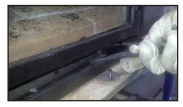
Figure 11.2. Glass Clip Tool Location
