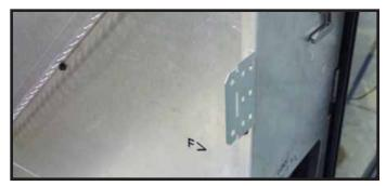
Figure 6.4 Nailing Tab Bent Out for Installation
