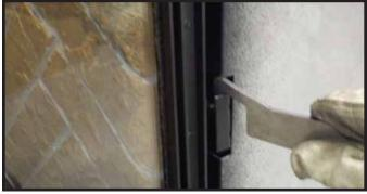
Figure 11.7. Securing Side Glass Clips
