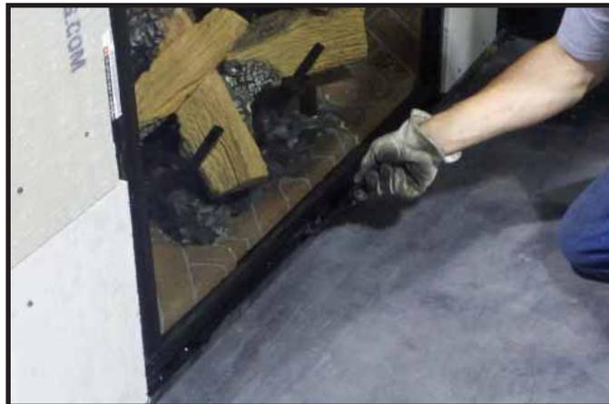
Figure 11.8. Securing Bottom Glass Clips
