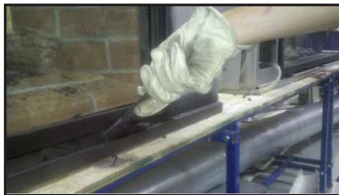
Figure 11.3. Inserting Glass Clip Tool
