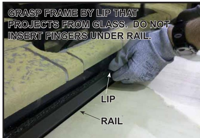
Figure 11.6. Installing Glass
