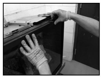
Figure 11.3 Release Glass Latches One at a Time
