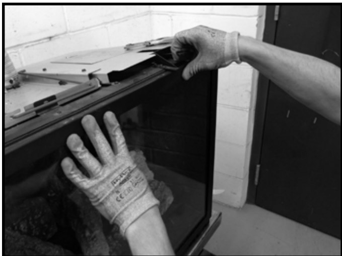
Figure 4.3 Release Glass Latches One at a Time
