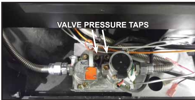
Figure 9.1. Valve Pressure Taps.
