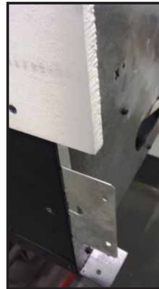
Figure 6.3 Nailing Tabs Installation Position
