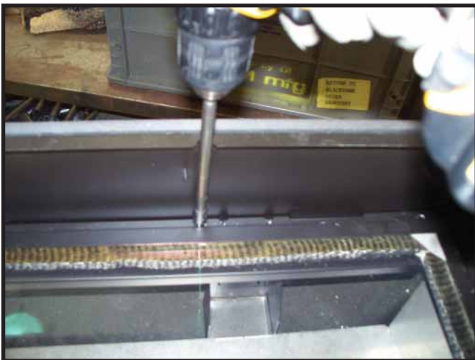
Figure 9.4. Gas and Electrical Access - Remove Glass Window
