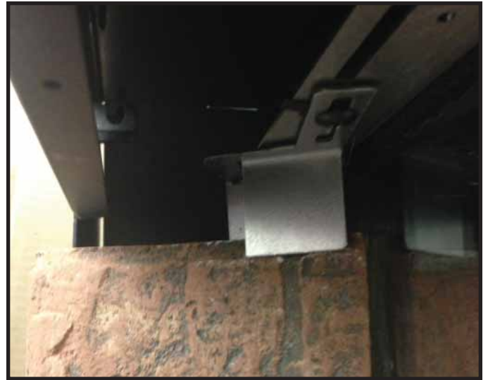
Figure 14.26 Side Refractory Brackets
