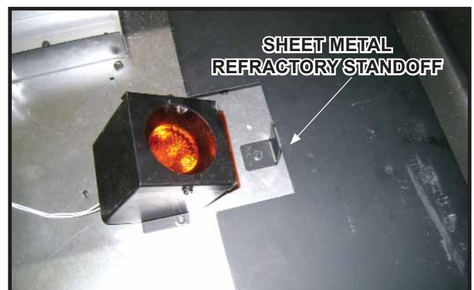
Figure 14.13 Accent Light Bulb Installation Completed
