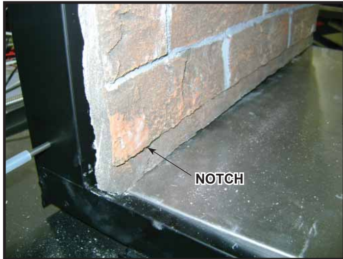
Figure 14.14 Notched End of Side Refractory
