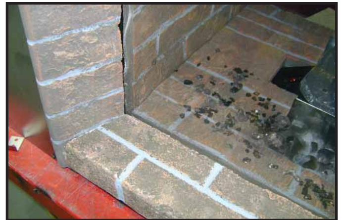
Figure 14.27 Outer Hearth Installation
