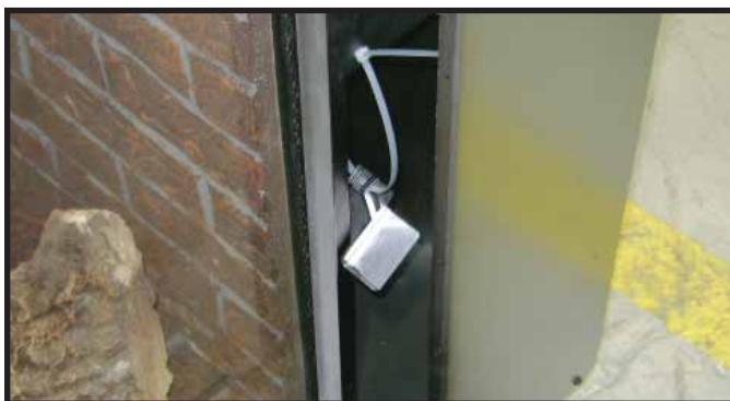
Figure 14.24 Shipping Location of Refractory Brackets
