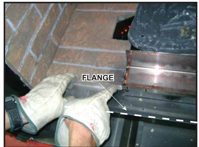
Figure 14.17 Positioning Left and Right Middle Base Refractory
