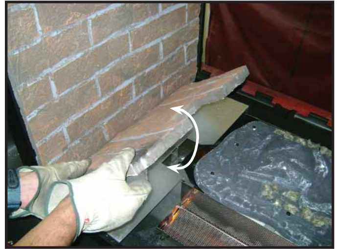
Figure 14.16 Positioning Inner Bottom Refractory
