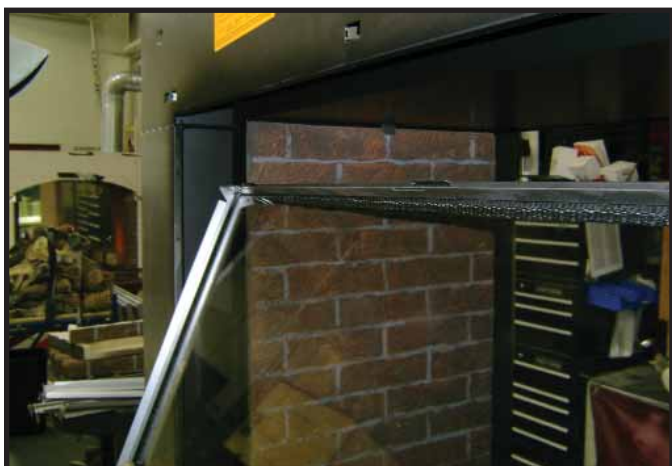
Figure 14.2 Initial Positioning of Frame into Opening.
