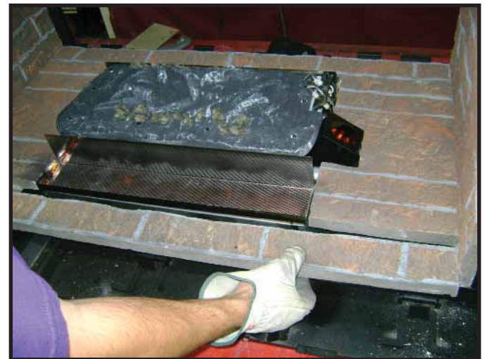
Figure 14.18 Positioning Outer Bottom Refractory.
