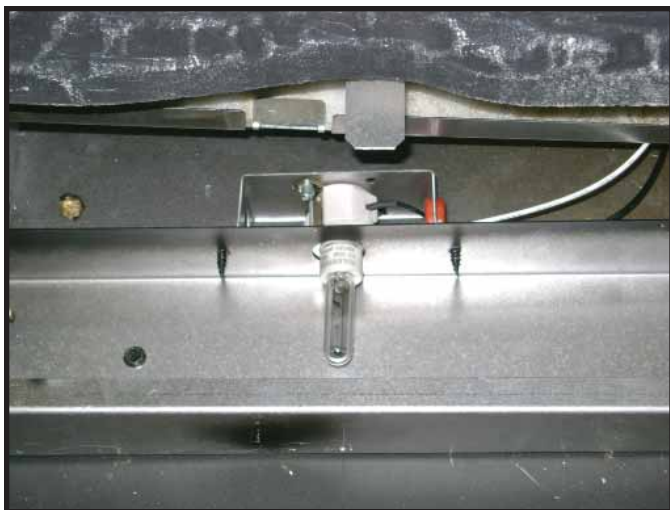
Figure 14.10 Ember Light Bulb Installed
