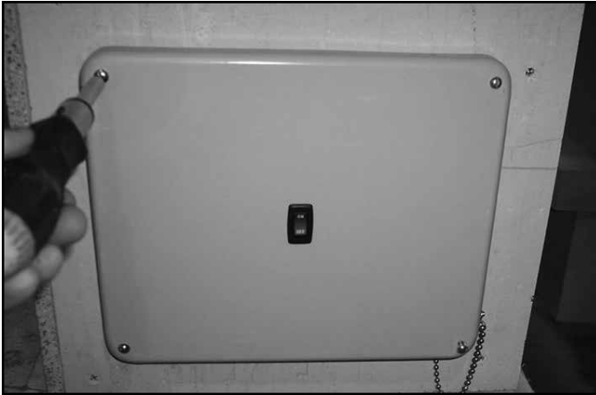
Figure 5.1 Remove Control Cover
