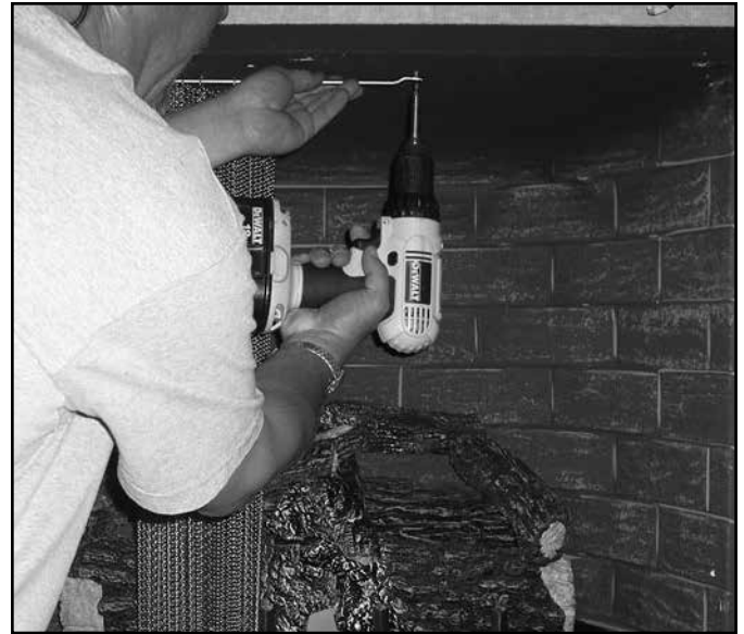
Figure 8.17 Fasten Screen Rod to Firebox Top
