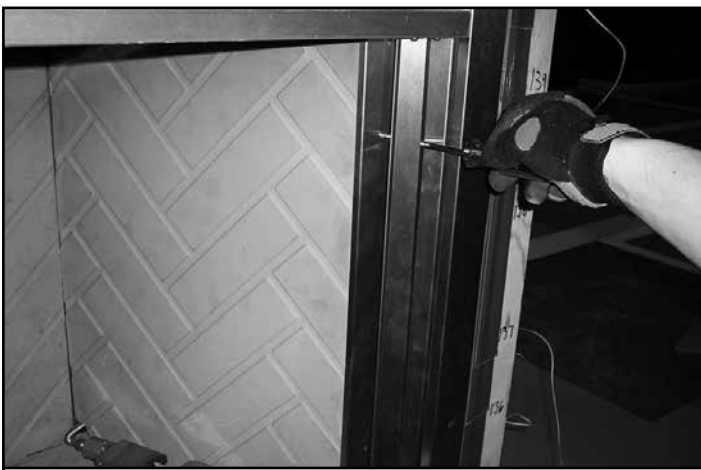
Figure 12.3 Loosen Refractory Retaining Strip
