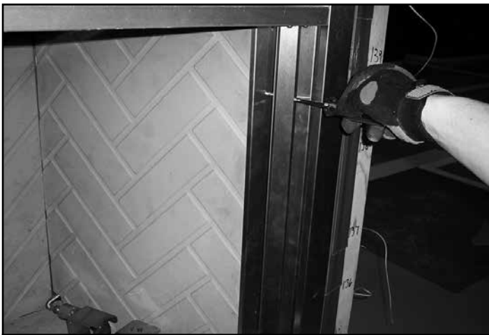
Figure 6.3 Loosen Refractory Retaining Strip
