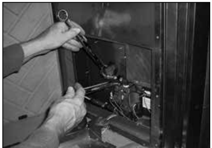
Figure 12.6 Turn off Gas Valve
