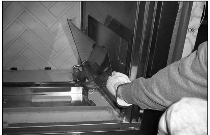
Figure 12.4 Remove Valve Access Panel
