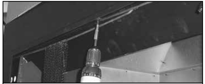
Figure 3.8 Removing the Screen Rods
