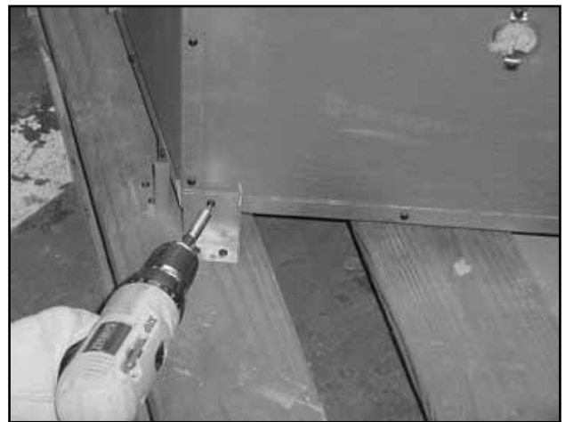
Figure 3.11 Removing Shipping Brackets
