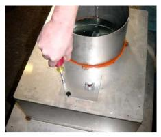
Route the electrical line through the romex clamp and attach the 120v wiring as detailed in the wiring diagram below. After the cover is replaced, tighten the clamp to secure the wiring.
