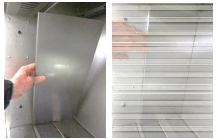
Install the inner glass panes before installing the end firebacks (NOTE: Remove the magnets before glass installation). The end fireback has angled top. Place the fireback with the slope facing outwards.
