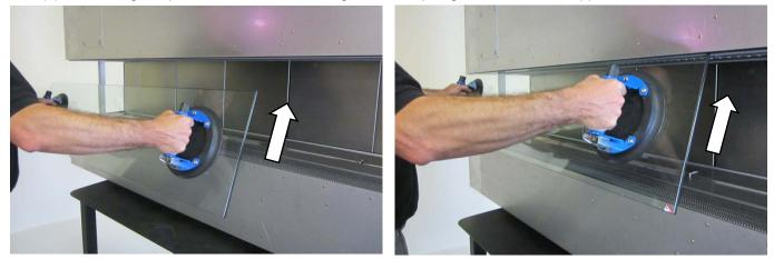
(c) Swing the lower edge of the glass pane inwards until the lower edge can insert into the lower slot.
