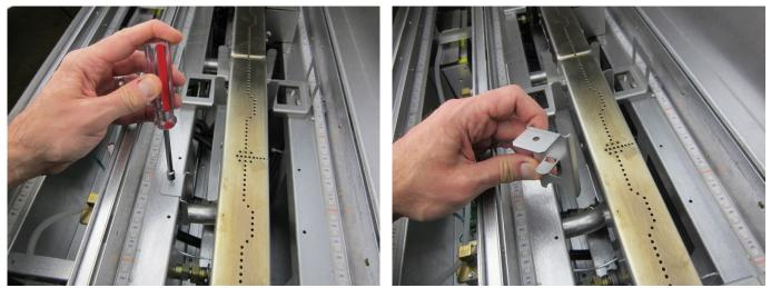
Lift the burner up and out of the fireplace. Remove the burner supports.
