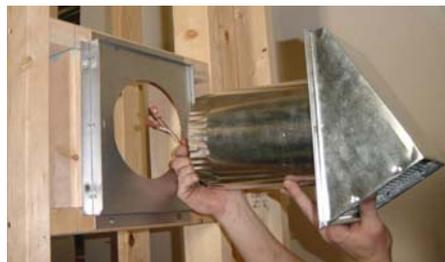
Secure the intake damper to the intake damper plate.
