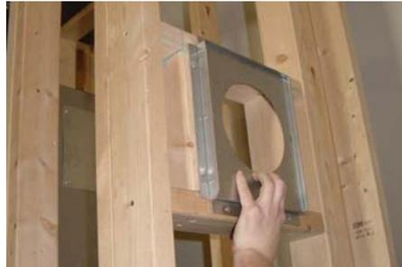
Slide the intake damper into place.
