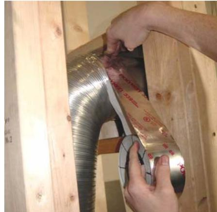
Route the flex duct to the fireplace air intake. Connect the wires from the air intake damper to the wires from the fireplace.
