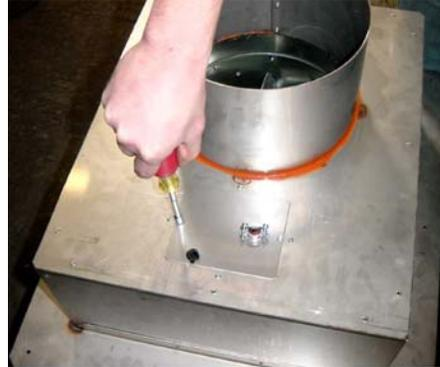
Route the electrical line through the romex clamp and attach the 120v wiring as detailed in the wiring diagram below. After the cover is replaced, tighten the clamp to secure the wiring.
