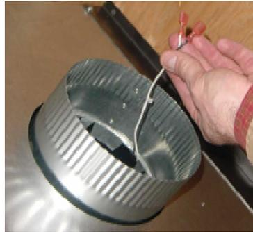
The intake damper requires a framed opening that is 8" (203mm) wide by 9" (229mm) tall. Secure the intake damper plate to the framing.
