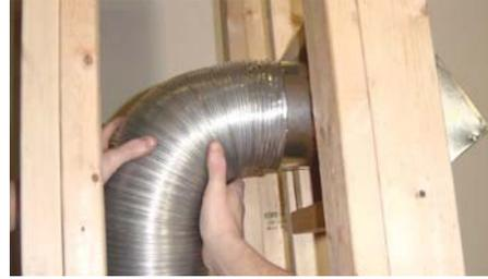
Secure the flex duct to the intake damper with two screws
