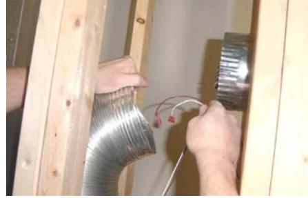
Slide the flex duct into place.
